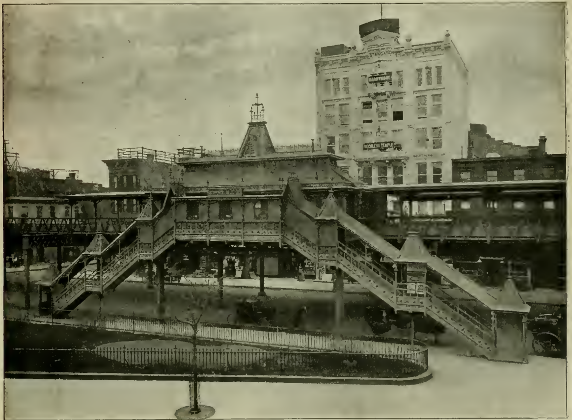
Fig. 1. THIRTY-THIRD STREET STATION, SIXTH AVENUE LINE.
